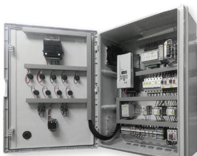
Example of installation of control equipment and accessories
